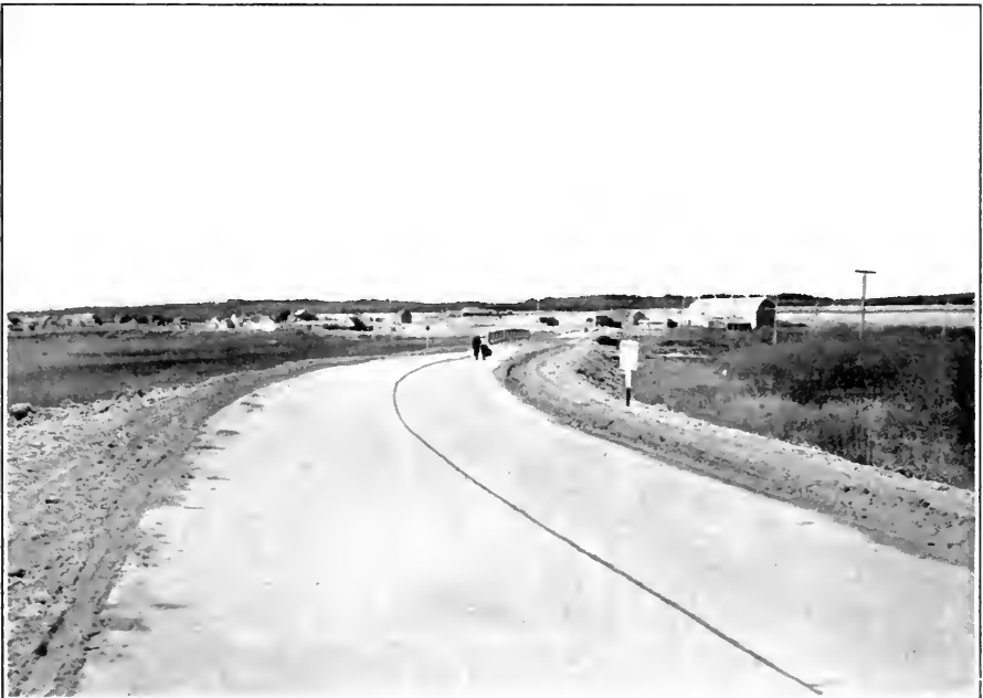
Concrete Pavement, Highway No. 67 at Porcupine
